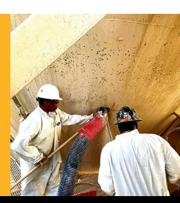
Using cutting-edge equipment like the Cardox CO2 System and the SiloWhip System, we safely clean storage vessels without human entry. These services not only enhance the operational efficiency and safety of storage systems but also comply with environmental standards, making them essential for industries like manufacturing and mining.
