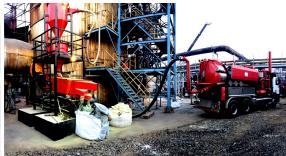
Special barriers are constructed inside convertors for personnel movements while vacuuming to avoid catalyst damage. Vacuumation suction pressure and catalyst velocity are also carefully controlled by our team of experts to avoid catalyst breakage. In addition, our team ensures that all ceramic ball layers are vacuumed separately from the catalyst.
