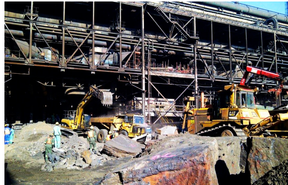
FURNACE DEMOLITION SERVICES
