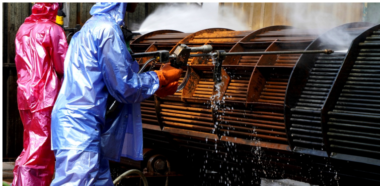
HP & UHP WATER BLASTING
