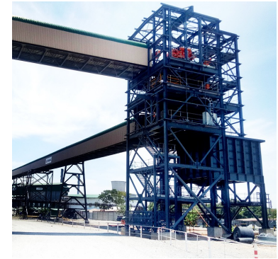
STRUCTURAL, MECHANICAL, PIPING, & PLATEWORK (SMPP)
