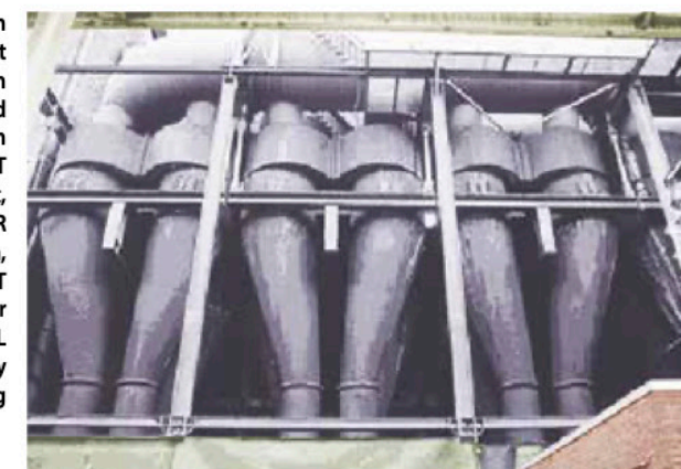
Dust collection cyclones for blast furnaces are effectively protected with combined linings
