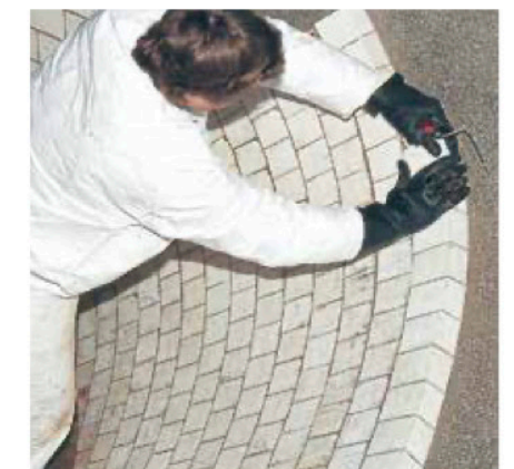
Kalenborn service solves wear problems on site
