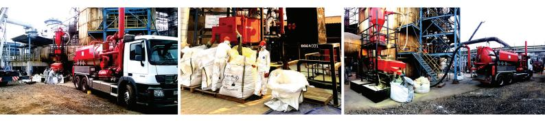
Special barriers are constructed inside convertors for personnel movements while vacuuming to avoid catalyst damage. Vacuumation suction pressure and catalyst velocity are also carefully controlled by our team of experts to avoid catalyst breakage. In addition, our team ensures that all ceramic ball layers are vacuumed separately from the catalyst.
